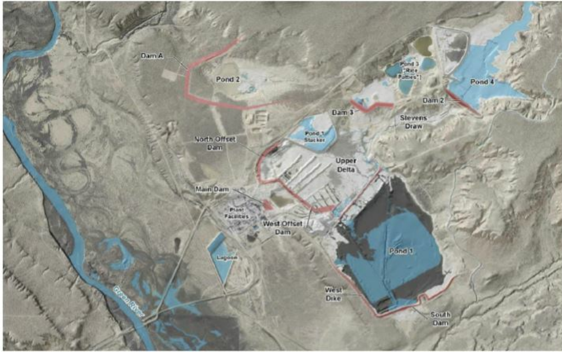
Source: Barr- Ciner-2020_Dam-Safety-Report_20210224-signed.pdf Figure 17.1 Şişecam Tailings Impoundments and Evaporative Ponds
